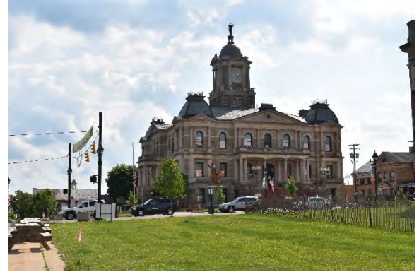
Figure 14 Harrison County Courthouse
