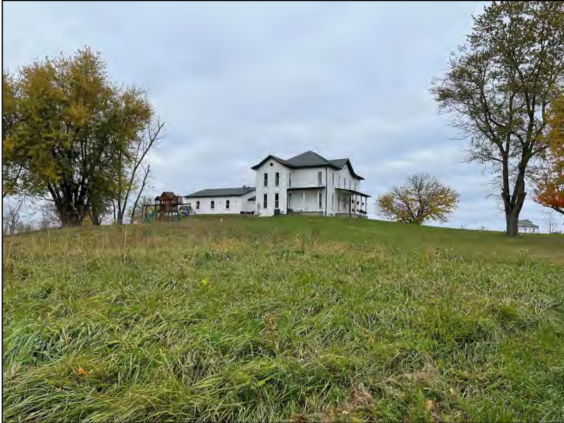
Figure 6: Overview of McLaughlin House Looking WNW
